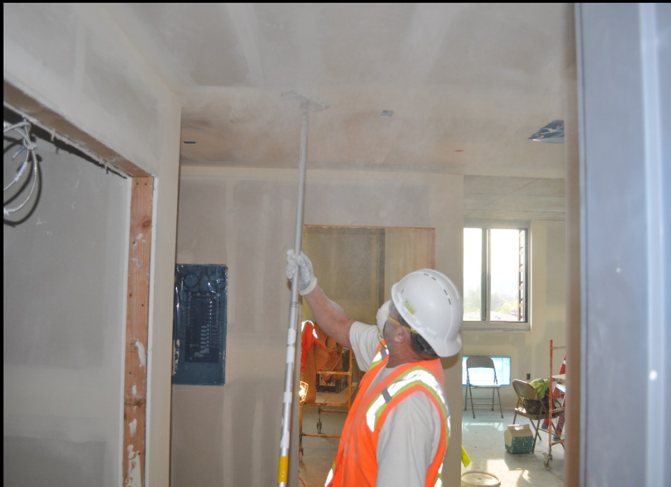
Drywall sanding 10 th floor
