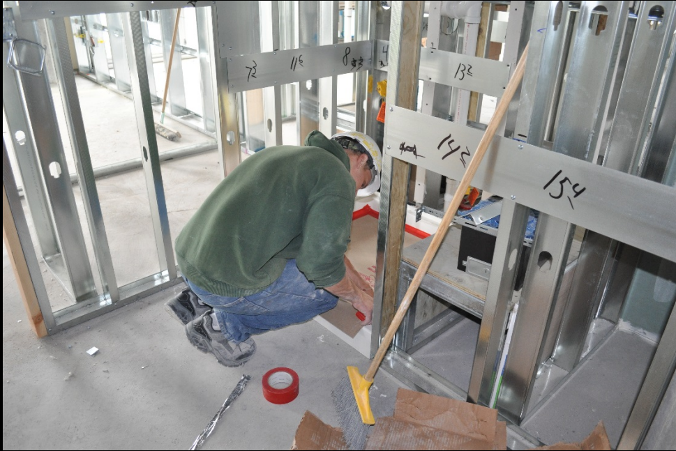
Installing shower pan protection 11 th floor
